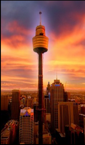
CENTER POINT TOWER , SYDNEY HAS RECORDED MORE THAN 40 STRIKES SINCE NOVEMBER 1995
