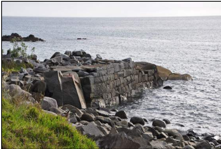
Fig. 8.2. This disused stone jetty at Paritu, northern Coromandel Peninsula, is made of Coromandel Granite blocks that were shipped out from here to many parts of New Zealand for use in many public buildings. Photographer Bruce Hayward.
