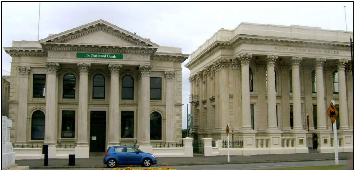
Fig. 15.12. Thirty million year-old Oamaru Limestone has been quarried for building stone for over 150 yrs and used in prominent stone buildings all around New Zealand and even in a few buildings overseas. Not surprisingly the best assemblage of Oamaru Stone buildings occur in Oamaru itself and include the National Bank (1871) and former Bank of New South Wales (1884) buildings in South Thames St. Photographer Bruce Hayward.
