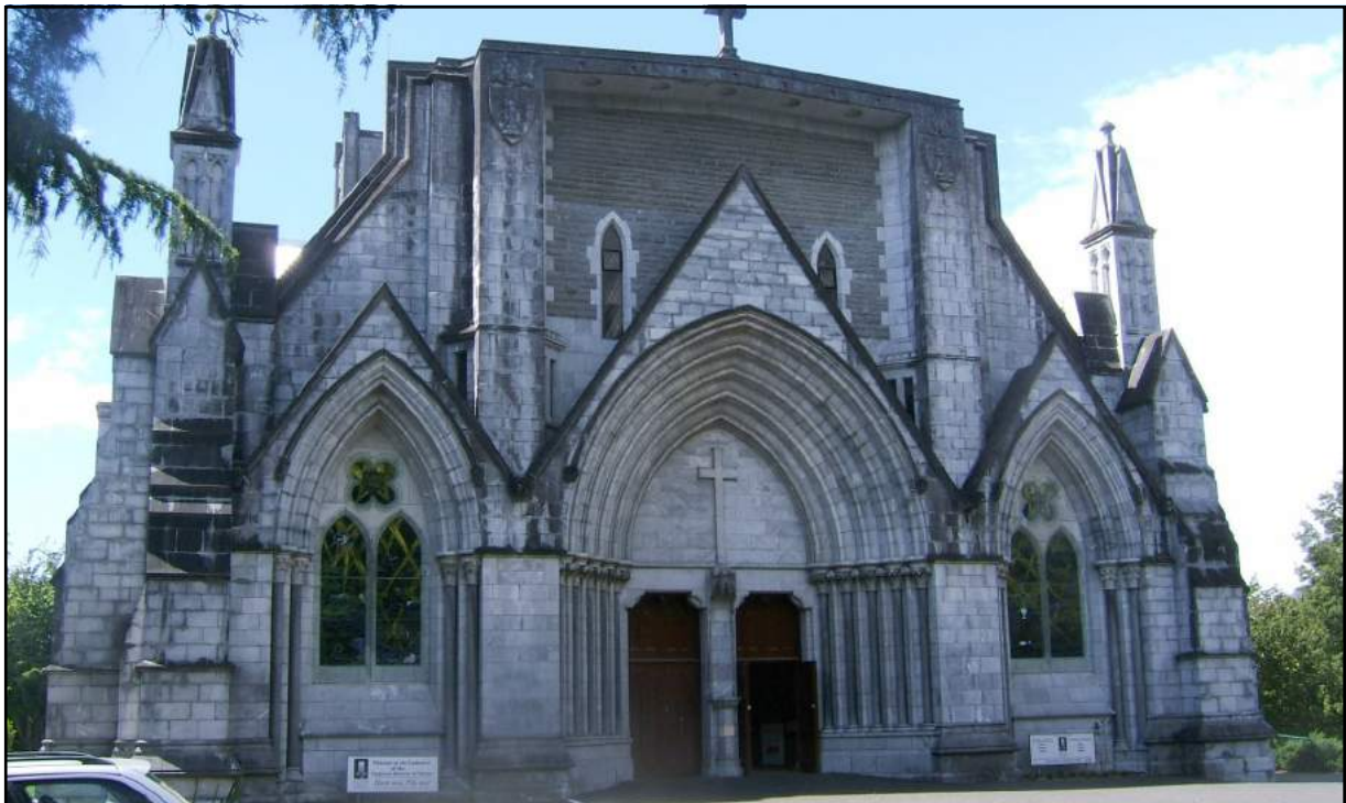
Fig. 21.4. Christ Church Cathedral, Nelson, is made of Arthur Marble (building stone name Kairuru Marble) extracted from near the top of Takaka Hill. Photographer Bruce Hayward.
