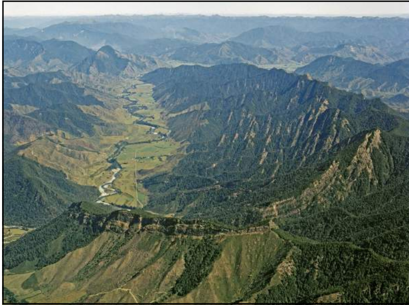
Fig. 20.7. Part of the Buller River runs down the eroded axis of the Longford Anticline near Murchison. The syncline was formed by strong tectonic compression during the last 5 myrs. Photographer Lloyd Homer, GNS Science.
