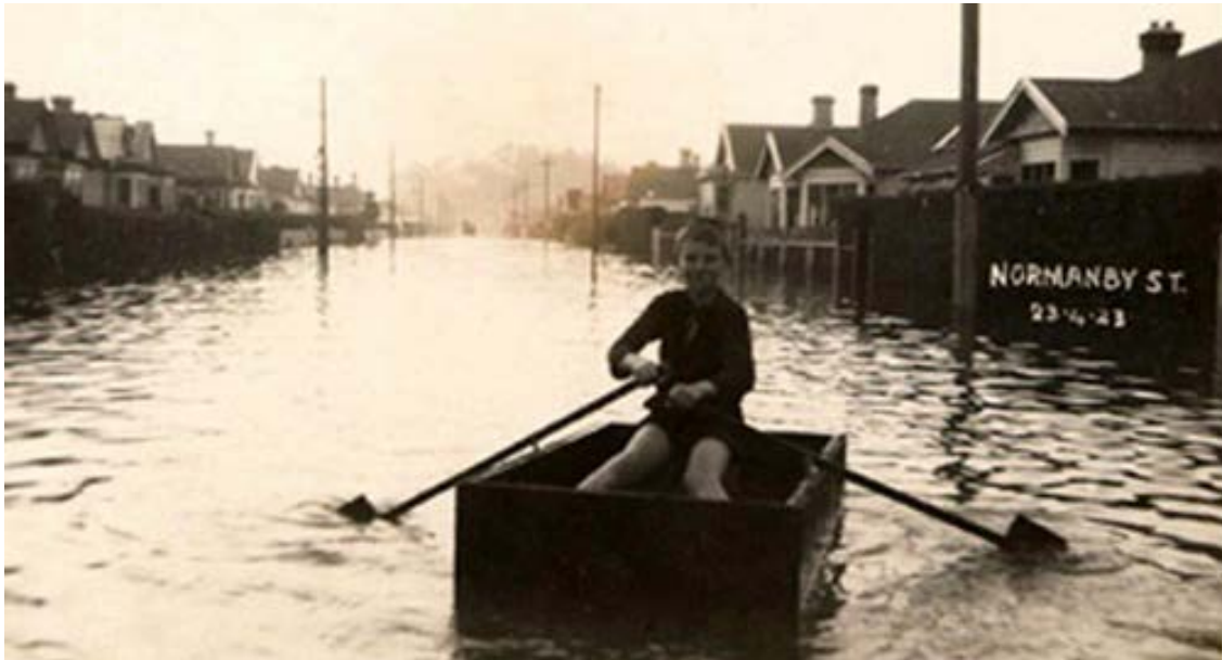
Figure 28. Ponding of surface water at south end of Normanby Street, April 1923, following heavy rainfall. This area was not badly affected in the June 2015 flood. Source: Otago Daily Times.
