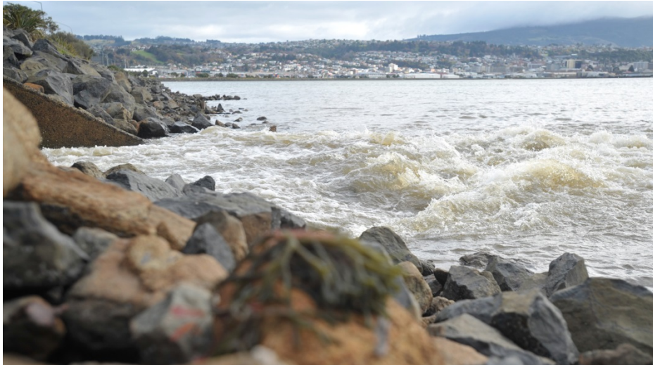
Figure 14. Stormwater outflow to Otago Harbour, near the intersection of Orari Street and Portsmouth Drive, June 2015. Source: Otago Daily Times.
